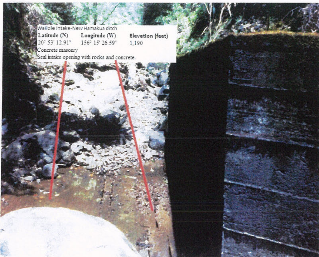
Photo 3 (above): Wailole at New Hamakua Ditch (NH-23)
